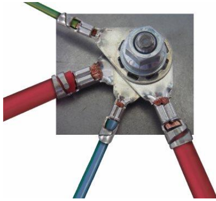
Typical single point (star) grounding
